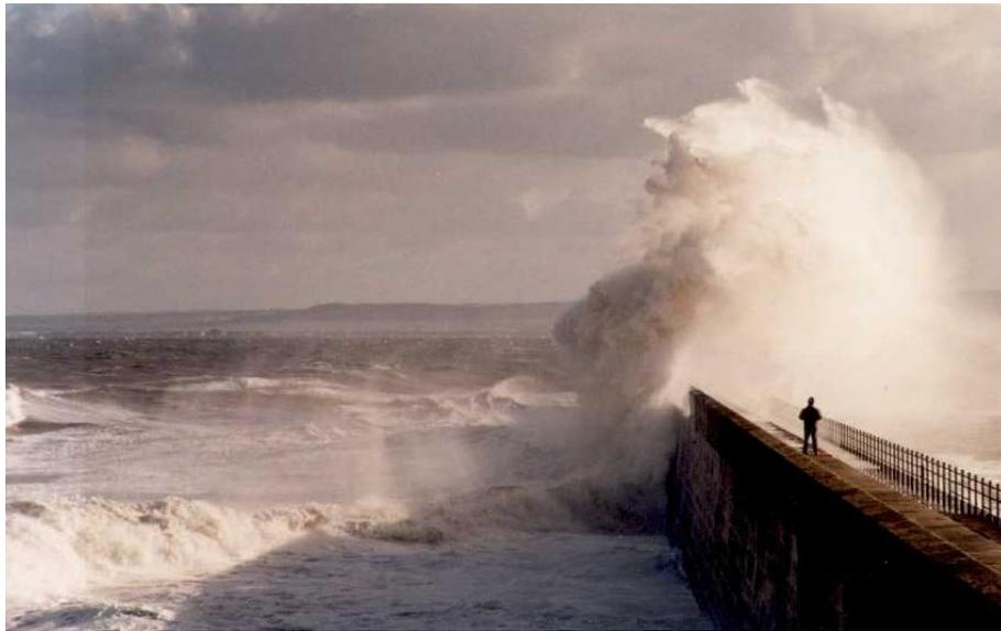
Figure 1: Violent wave overtopping occurs when waves break against sea walls throwing water and spray over the top.
