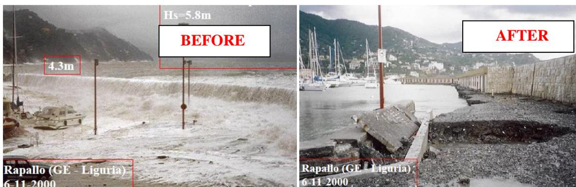
Figure 31: Left: Harbour Rapallo during wave attack on the 6th Nov 2000. Right: Damaged harbour Rapallo after the wave attack.
