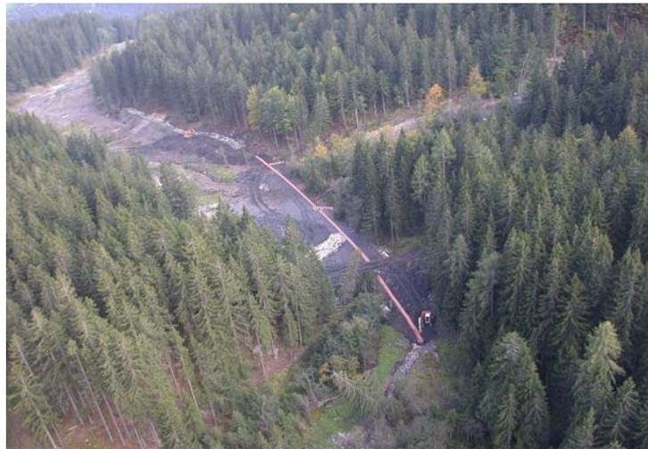
Figure 12. The Macesnik Landslide in its upper part showing the execution of surface drainage works in 2004 (from Mikos et al., *Natural Hazards and Earth System Sciences*, Vol. 5, No. 6, 2005, p. 952).
