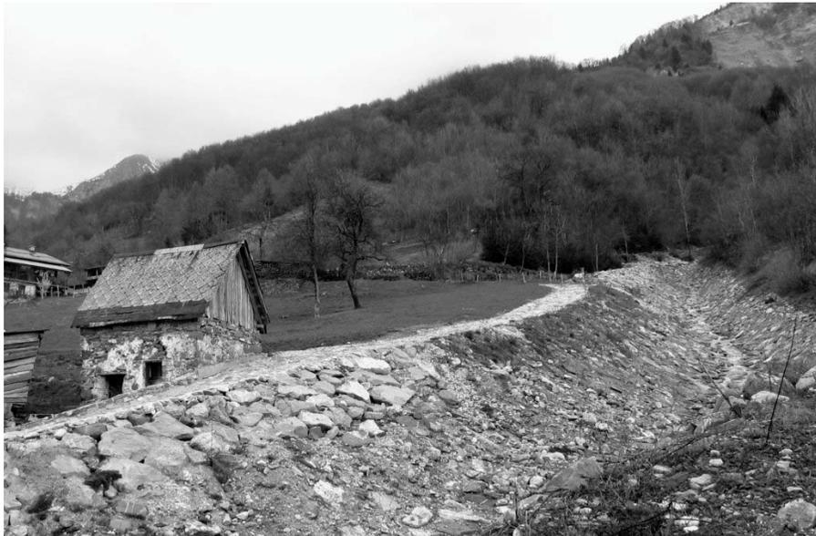
Figure 9. The enlarged parabolic channel of the Brusnik Stream in Koseč was protected using rip-rap and as such in 2002 it was conveying more than 20 debris flows with the magnitude from around  $100 \text{ m}^3$  to around  $1000 \text{ m}^3$ .
