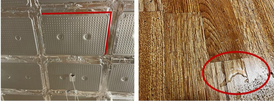
Figure 6.22: PCM leakage due to volume expansion dropping from the ceiling on the floor.
