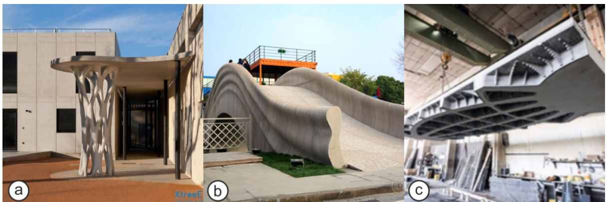
Figure 14: Prefabricated 3DCP: (a) column from Xtree, (b) bridge from Tsinghua University, and (c) slab from TU Graz
