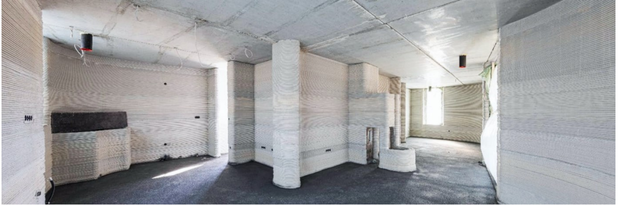
Figure 16: The interior of the 3DCP house in Germany [21]
