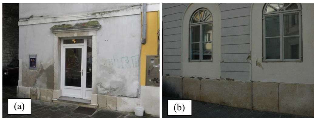
Figure 61: Condition of buildings after the impact caused by the sea flood in November 2019 (0.4m flood depth): (a) Obzidina ulica 2; (b) Tartini Square 2;
