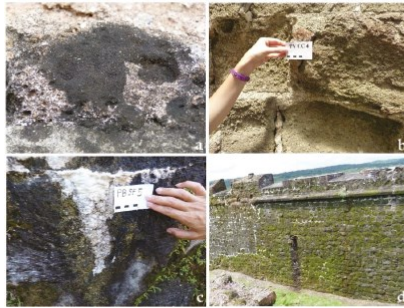
Figure 9: Pictures representing several deterioration processes observed at the sites. (a,b) at Panamá Viejo, (a) biological growth; (b) surface recession/material loss; (c) encrustation at Fort San Fernando (Portobelo); (d) biological growth at Fort San Lorenzo (Ciantelli et al., 2018)
