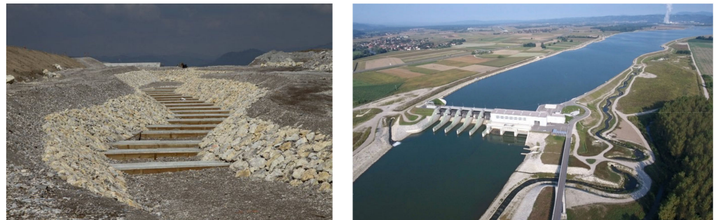
Figure 3. An exemplary fishway at HPP Brežice, Sava River.
