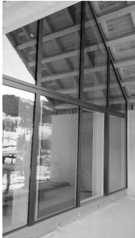
**Figure 1.** An example of window elements with a height of 5.8 m.
