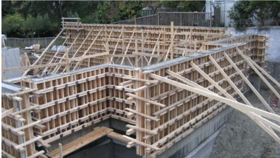
Figure 1: Example of Conventional formwork system[8]
