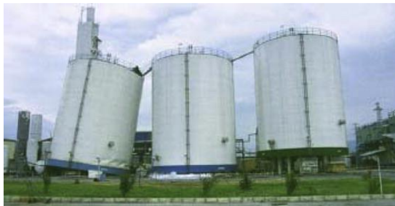
Fig. 1. View of the non-code-conforming elevated steel storage tank that collapsed during the earthquake [12].
